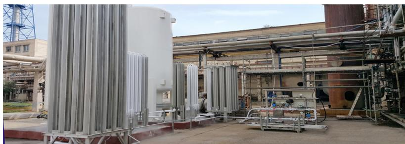
**Figure 4.** Test equipment including a mobile tank, vaporisers, fundamentals, regulation skid and flexible hoses.
