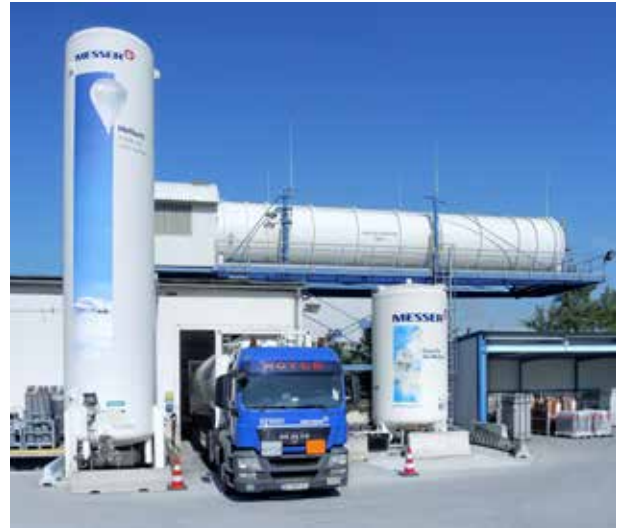
120'000 l horizontal tank container for liquid helium
