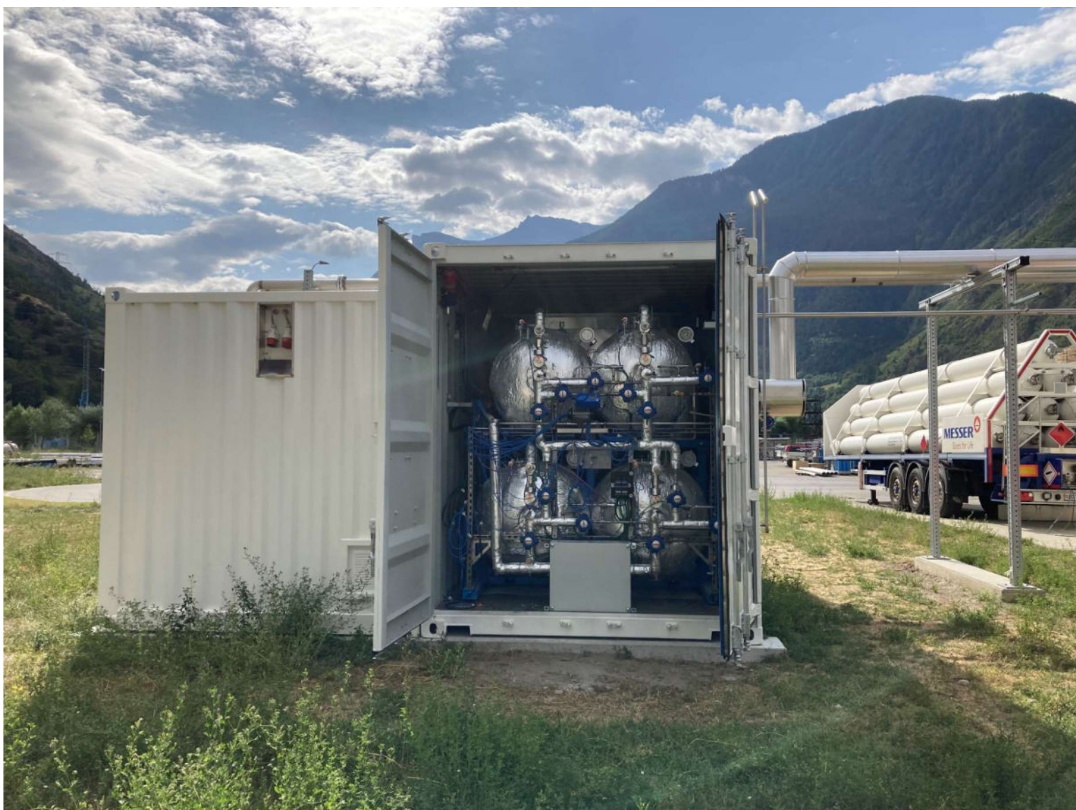
Thermal compressor for filling hydrogen trailers at the Visp site, Valais, Switzerland
